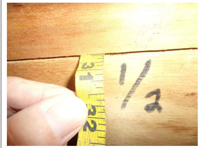
ROOF DECK THICKNESS – ½ inch plywood
