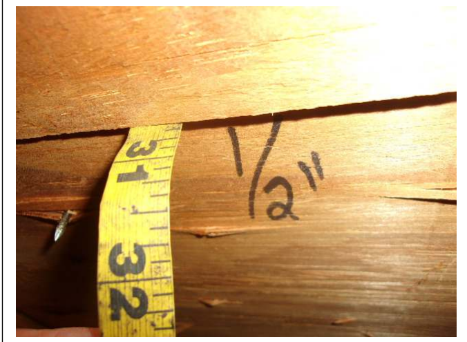
ROOF DECK THICKNESS – 1/2 inch plywood
