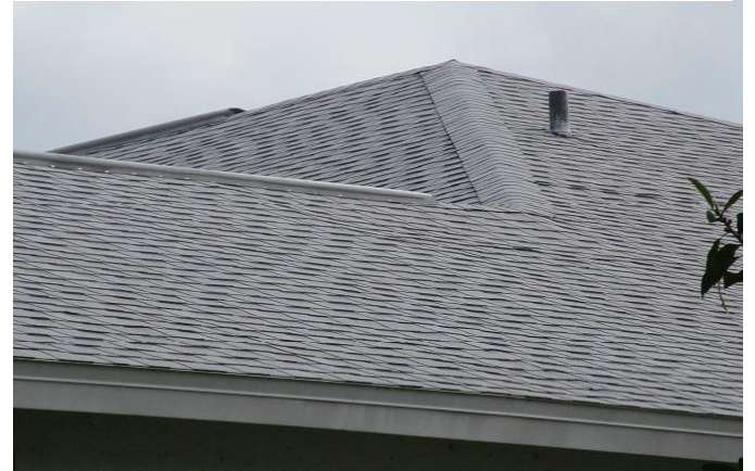
#2) roof covering: 2018 dimensional asphalt shingle HIP style roof PRBD2018-0848387 applied 8/13/2018
