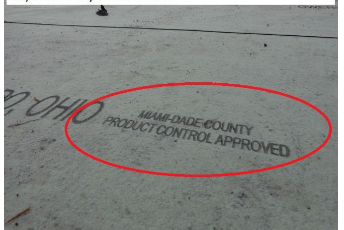
#6) secondary water barrier
