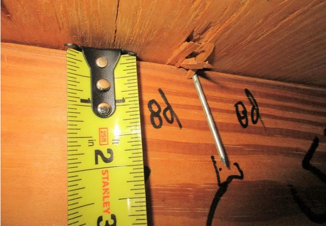
#3) roof deck attachment: 8d nails
