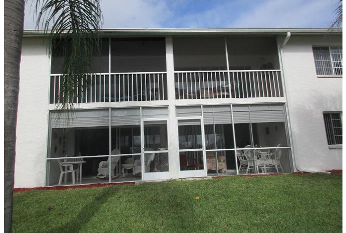
#7) opening protection: non impact sliders (some w/shutters)
