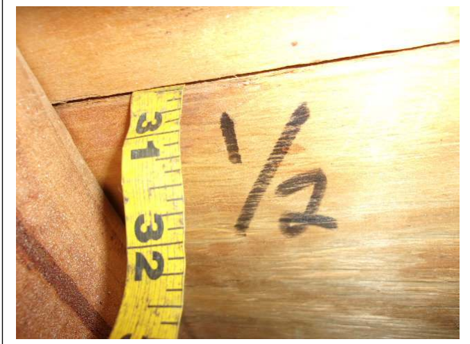
ROOF DECK THICKNESS – ½ inch plywood
