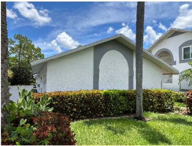
ROOF GEOMETRY – Gable / Other Roof Shape
