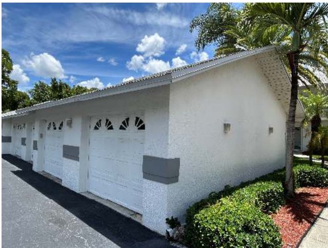
ROOF GEOMETRY – Gable / Other Roof Shape
