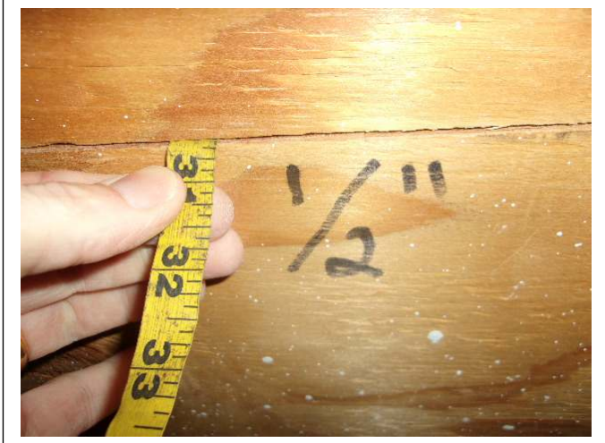
ROOF DECK THICKNESS – ½ inch plywood
