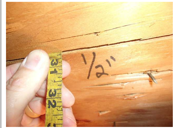
ROOF DECK THICKNESS – 1/2 inch plywood
