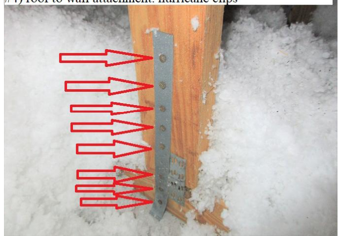
#4) roof to wall attachment: hurricane clips
