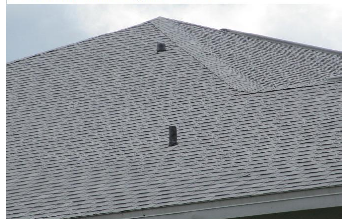
#2) roof covering: 2018 dimensional asphalt shingle HIP style roof PRBD2018-0848379 applied 8/13/2018
