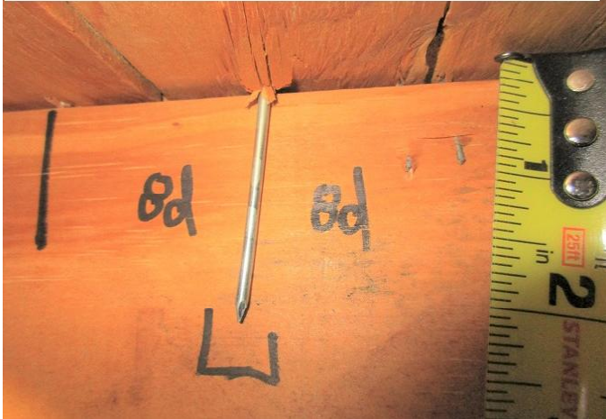
#3) roof deck attachment: 8d nails
