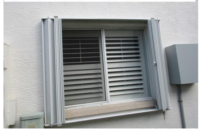
#7) opening protection: non impact windows- some with storm protection & most without storm protection
