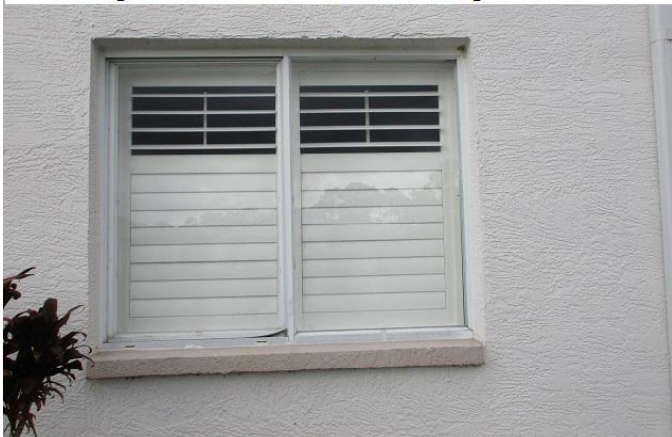
#7) opening protection: non impact windows- some with storm protection & most without storm protection
