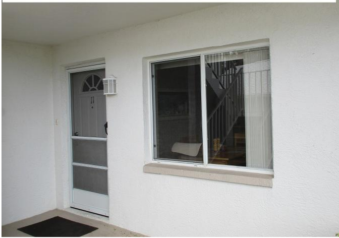
#7) opening protection: non impact front entrance
