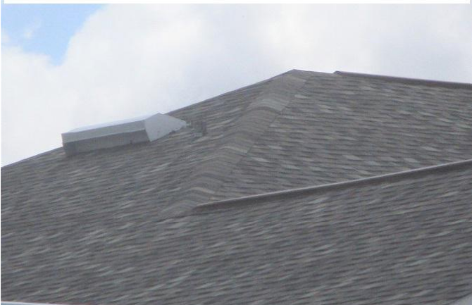
#2) roof covering: 2018 dimensional asphalt shingle HIP style roof PRBD2018-0424715 applied 4/11/2018
