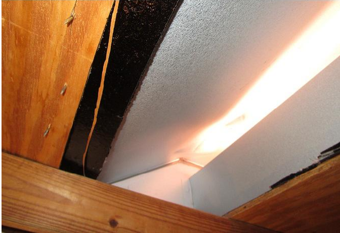
*secondary water barrier (resistance) as viewed from attic (off ridge vent)
