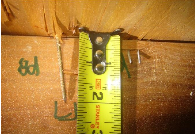
#3) roof deck attachment: 8d nails
