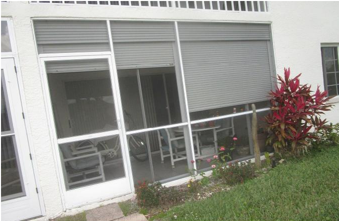
#7) opening protection: rear porches - non impact sliders, some w/roll down shutters
