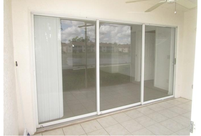
#7) opening protection: rear porch- non impact sliders
