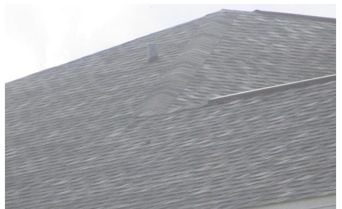
#2) roof covering: 2018 dimensional asphalt shingle HIP style roof PRBD2-018-0244720 applied 4/11/18
