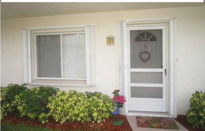
#7) opening protection: non impact windows (some w/protection) And non impact front entrances
