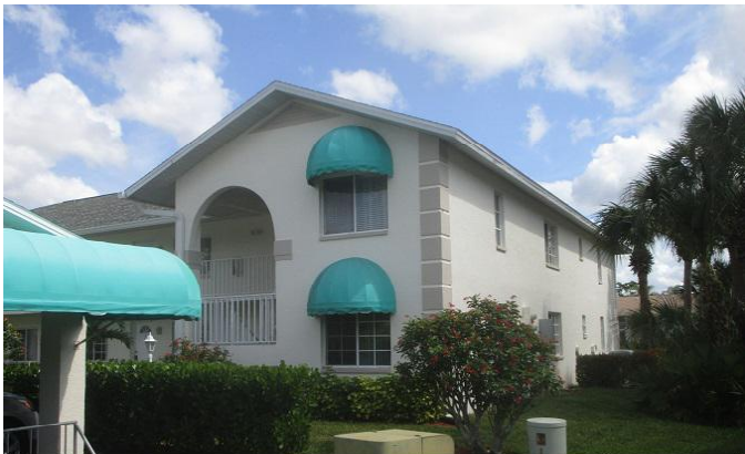
#5) roof geometry: HIP style roof *36' front gables vs 398' total roof perimeter or less than 10% **wall type construction: 95% reinforced masonry
