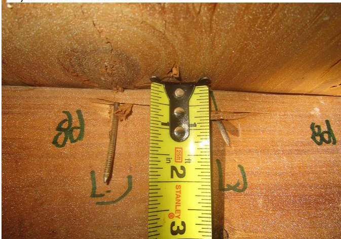
#3) roof deck attachment: 8d nails
