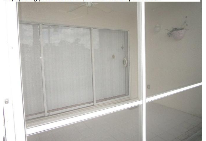
#7) opening protection: rear porches - non impact sliders
