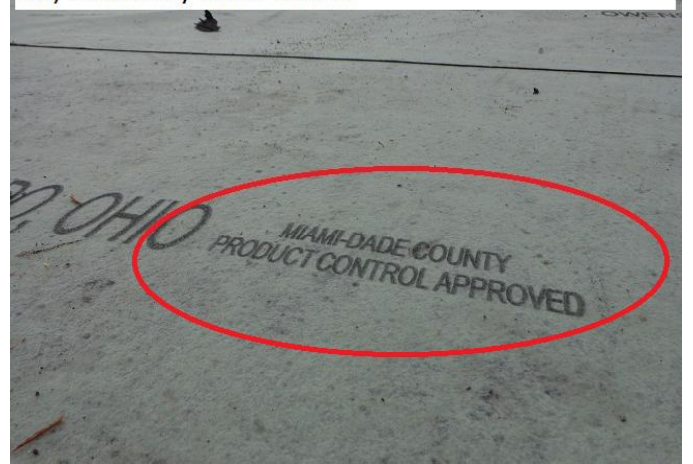
#6) secondary water barrier
