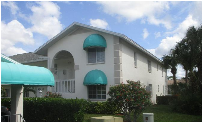
#5) roof geometry: HIP style roof *36' front gables vs 398' total roof perimeter or less than 10% **wall type construction: 95% reinforced masonry
