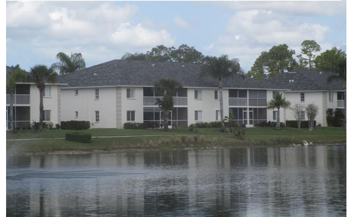
#5) roof geometry: HIP style roof **wall type construction: 95% reinforced masonry
