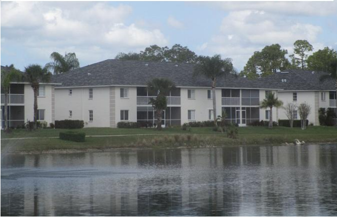
#5) roof geometry: HIP style roof
