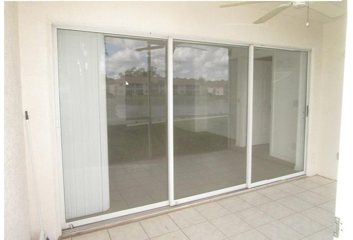
#7) opening protection: rear porch- non impact sliders
