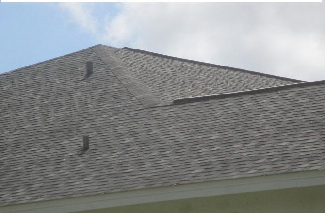
#2) roof covering: 2018 dimensional asphalt shingle HIP style roof PRBD2018-0424721 applied 4/11/2018
