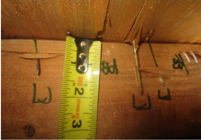
#3) roof deck attachment: 8d nails
