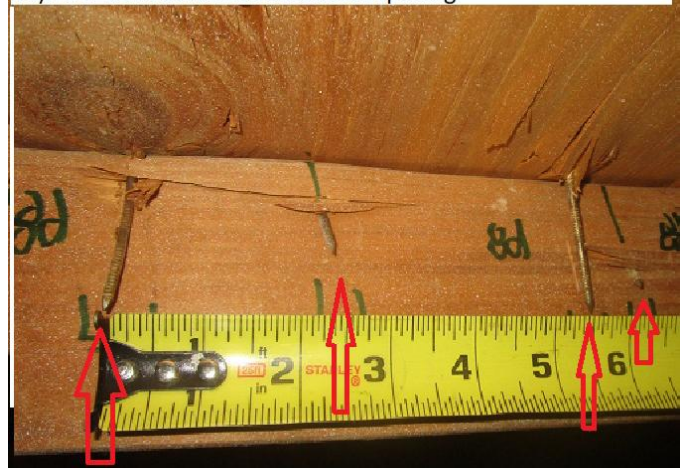
#3) roof deck attachment: 8d nail spacing
