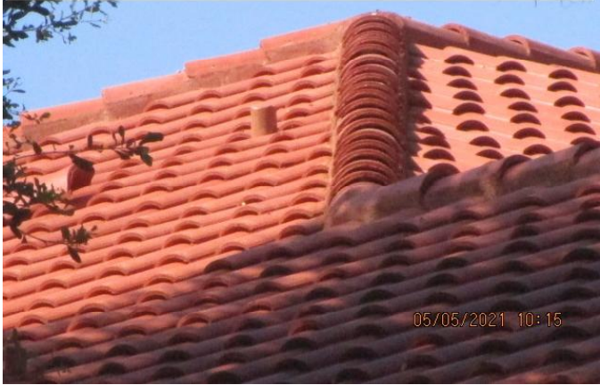
#2) roof covering: 2021 TILE "other" style roof PRBD2021-0206940 applied 2/18/2021
