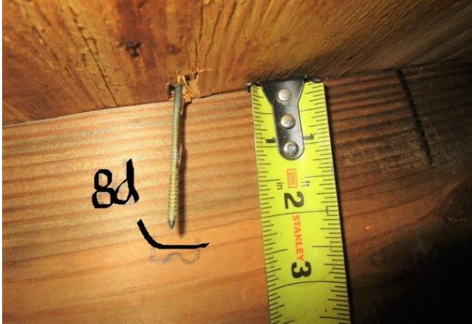
#3) roof deck attachment: 8d nails
