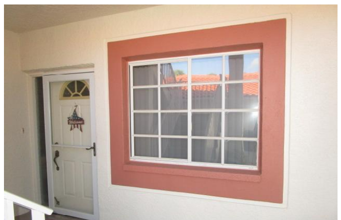
#7) opening protection: non impact windows (some w/hurricane protection)
