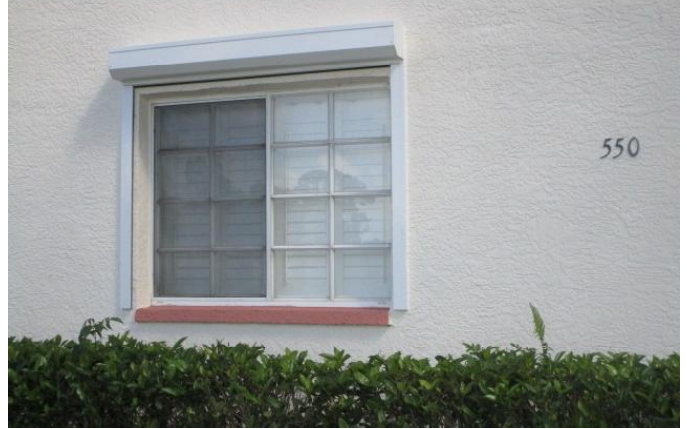
#7) opening protection: non impact windows (some with hurricane protection)
