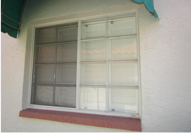
#7) opening protection: non impact windows
