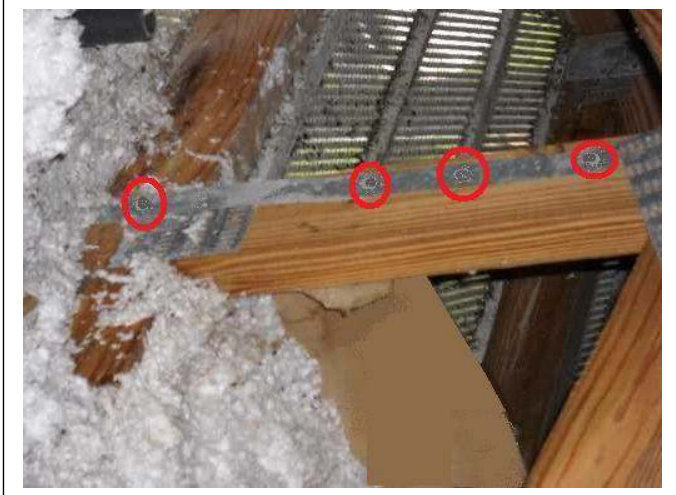
ROOF TO WALL ATTACHMENT – Properly installed Clips
