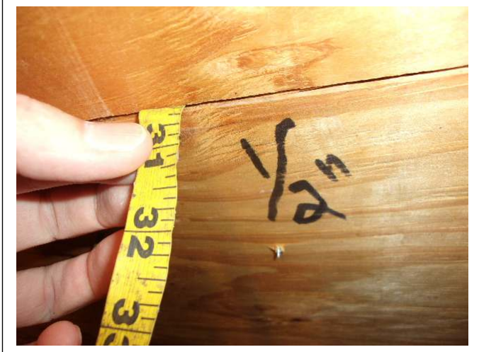
ROOF DECK THICKNESS – ½ inch plywood
