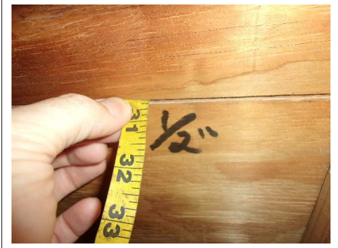
ROOF DECK THICKNESS – ½ inch plywood
