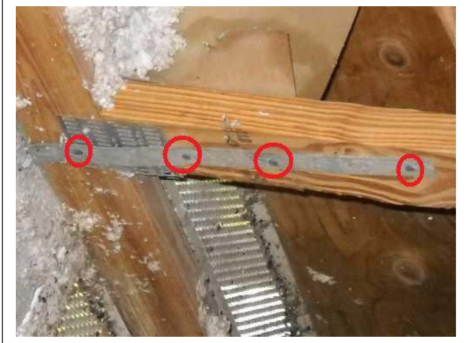
ROOF TO WALL ATTACHMENT – Properly installed Clips
